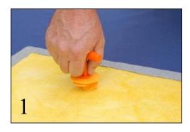
Screw Rotofast Snap-On Anchors into the back of the panel using the Rotofast driver tool.
