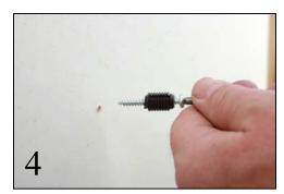
Screw ratchets to wall at marked locations. (#8 screws recommended)
