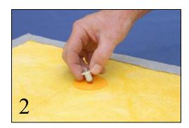
Insert marking plugs into the Snap-On anchors.
